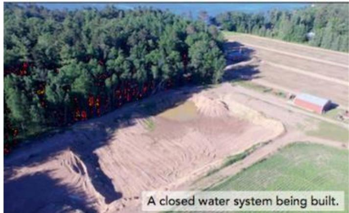
As part of a rejuvenation of his six-acre bog near Point O' Pines on Lac Courte Oreilles, Gary G. Jenson, owner of Castle Rock Cranberries LLC, has constructed a closed system and installed piping and pumps that will eliminate the need to discharge used water back into Lac Courte Oreilles. This closed system won't be placed into operation until new cranberry vines begin to produce fruit, a couple years from now.
